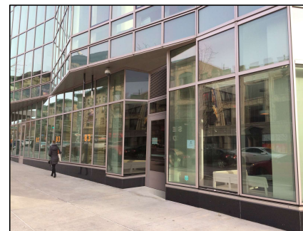
Image 7: Examples of Wind Control Measures for Building Entrances
