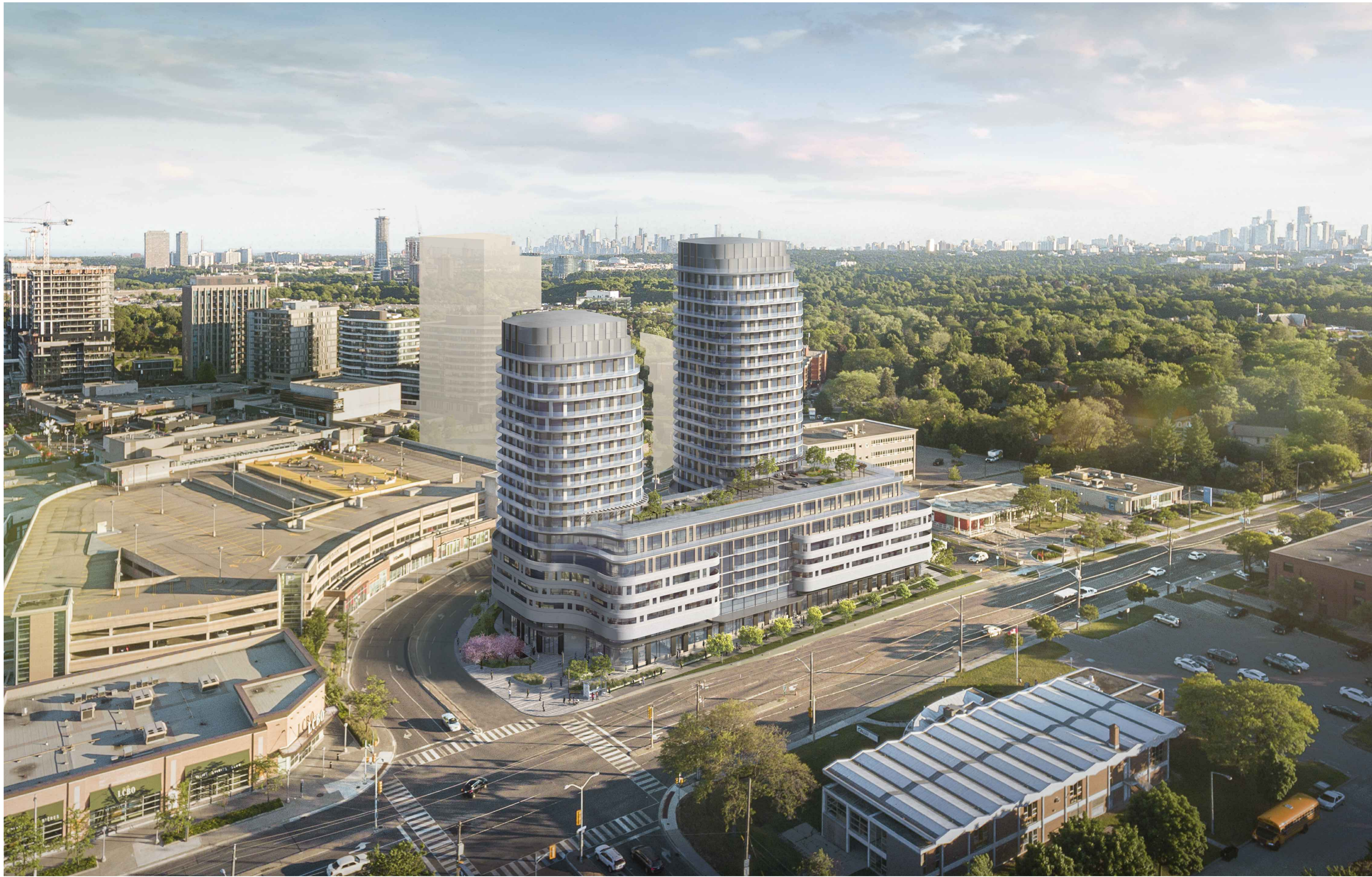
1 AERIAL VIEW SOUTH EAST 4406A
