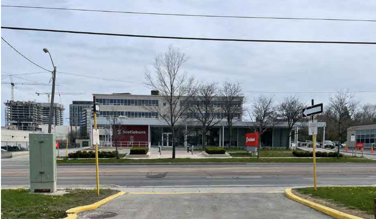
19. North elevation of 885 Lawrence Avenue East, visible from Lawrence Avenue East (ERA, May 2022).
