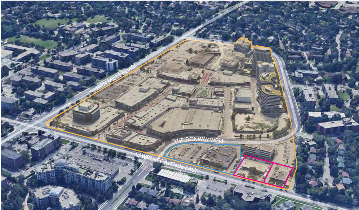
5. View of the surrounding neighbourhood context (Google Earth, 2022).
