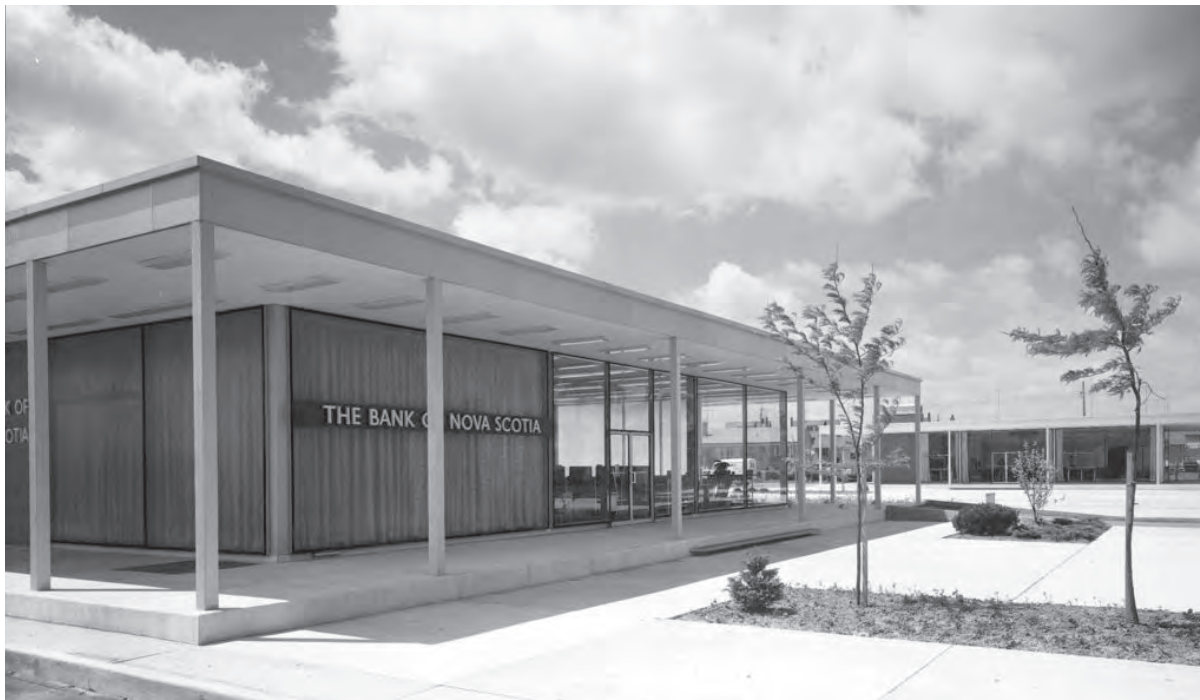
18. Exterior of the Bank of Nova Scotia after construction in 1957 (Panda Archives, 1957).
