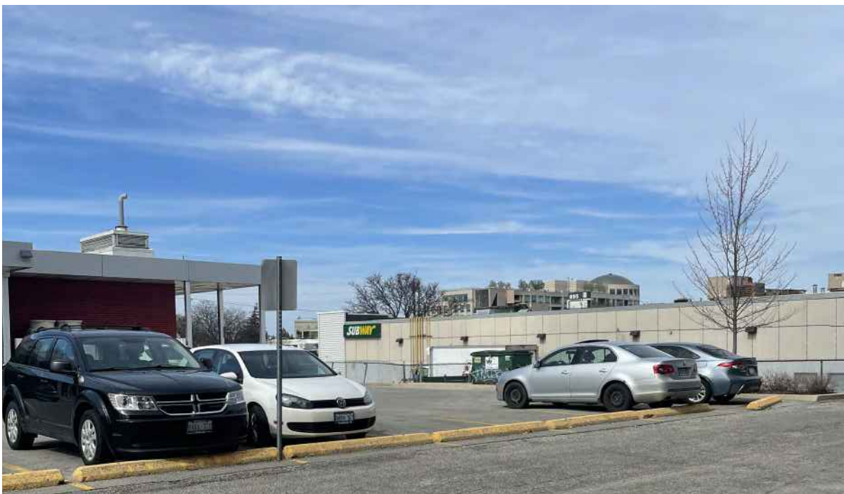
4. Partial view of the west elevation of the Site, from south parking lot (ERA, May 2022).
