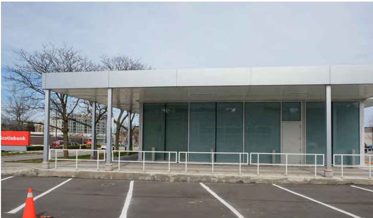
22. West elevation of 885 Lawrence Avenue East (ERA, May 2022).
