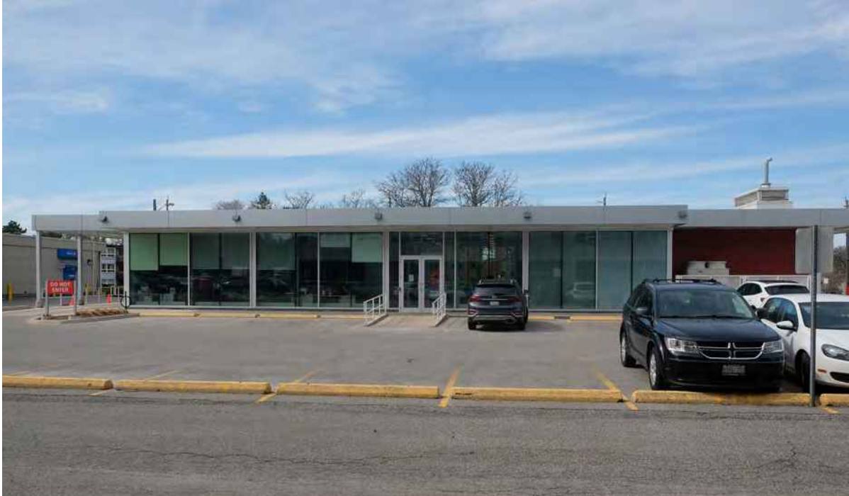
21. South elevation of 885 Lawrence Avenue East (ERA, May 2022).
