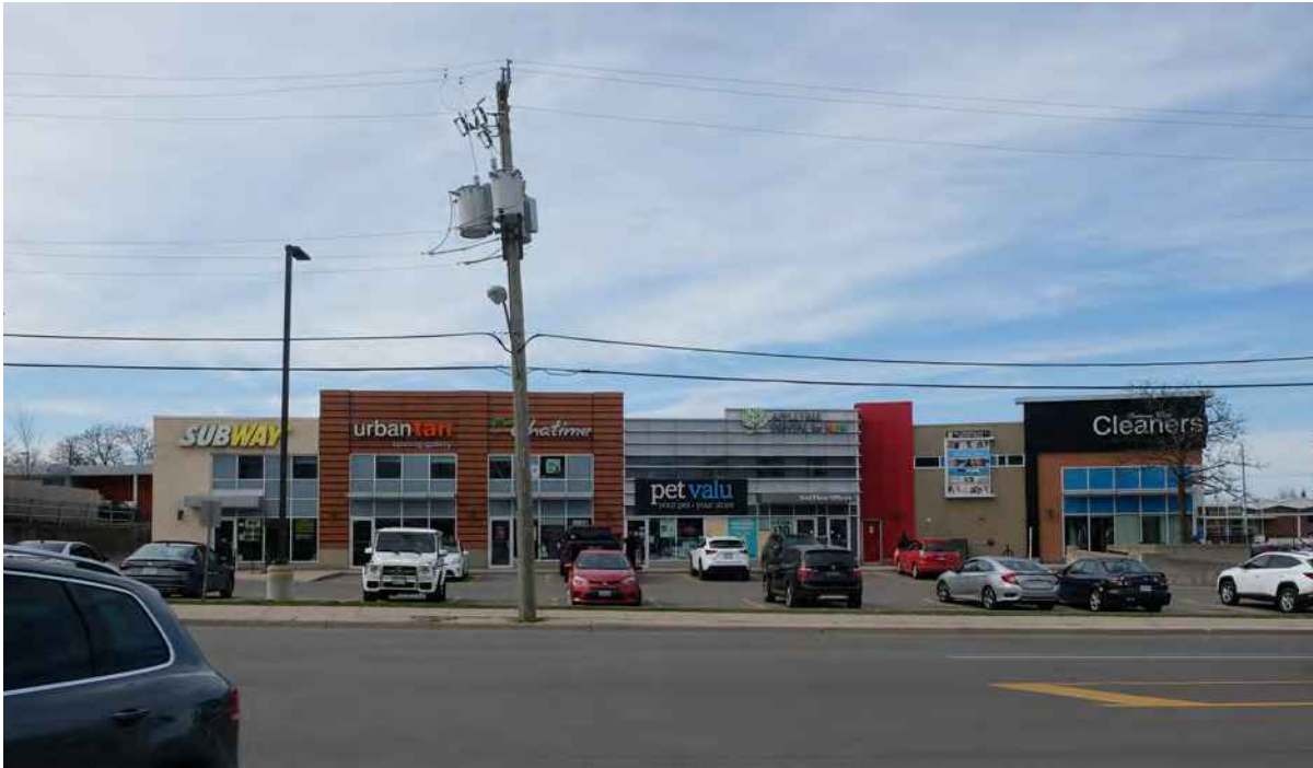
3. South elevation of the Site, also visible from The Donway West (ERA, May 2022).
